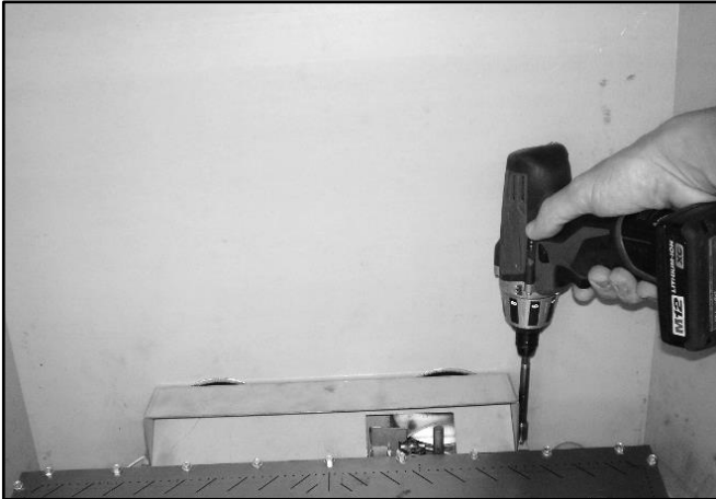
Step One: Remove Log Holder.
